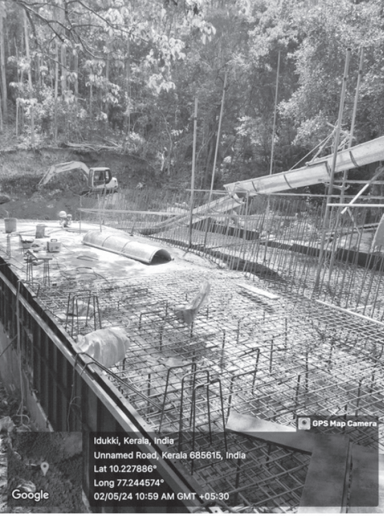
22.00 %: Concreting Image 6 of 7
