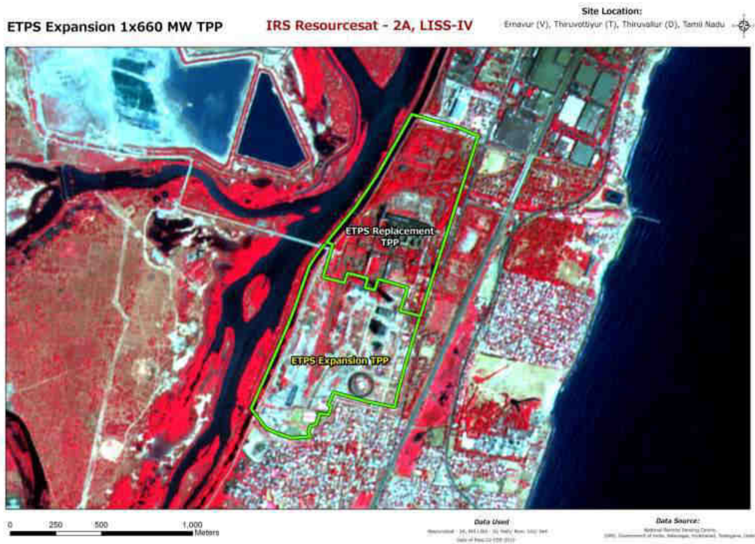
Figure 3.10: Satellite imagery of the project site
