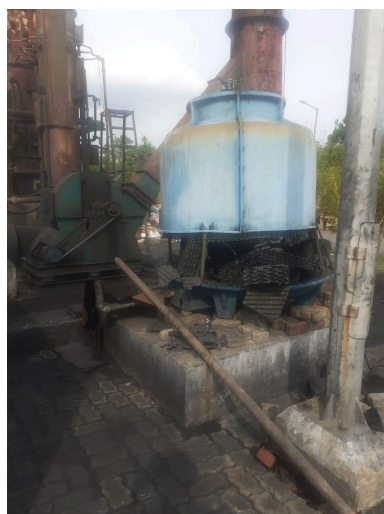
Fig 4: Damaged and non-functional air pollution control system
