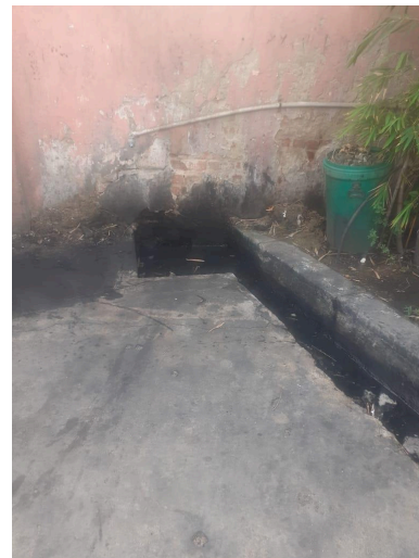
Fig 6: Untreated toxic leachate discharged directly into the drain
