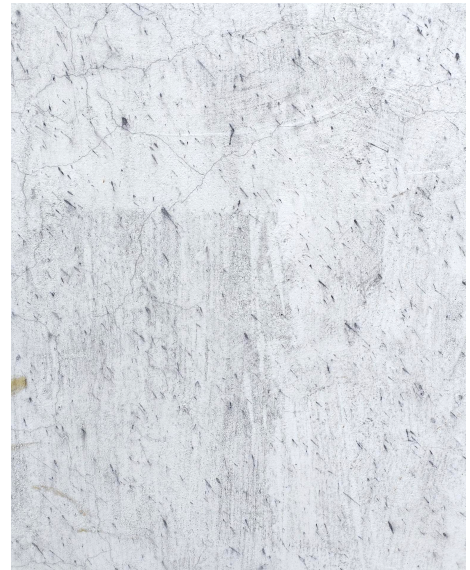
Fig 1: Deposition of black soot from the incinerator on the walls of the residences
