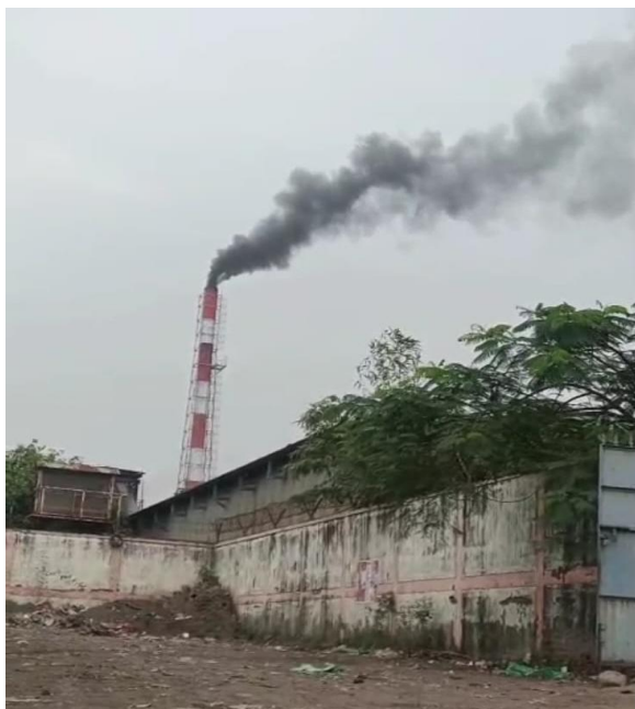
Figure 4: Toxic fumes emitted by the incinerator facility on Jan 10,2026
