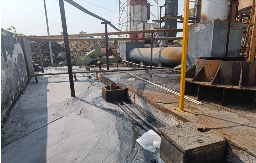
Figure 2: Toxic leachate overflowing from the effluent treatment plant
